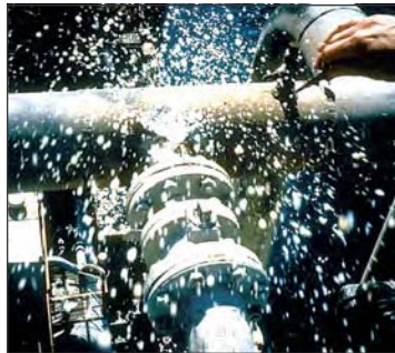
LEAKING PIPE
